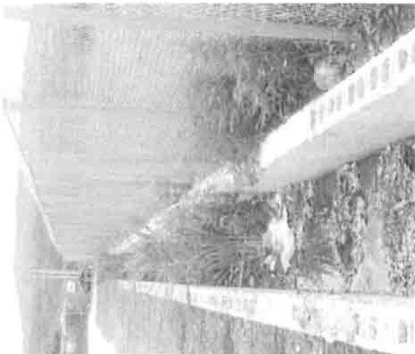
Figure 7: Showing one of the storm water drains on the campsite partially blocked by plants and debris.
