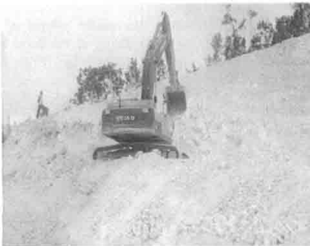
Figure 5: Showing excavator cutting bench near Phoenix Park, St. Ann.
