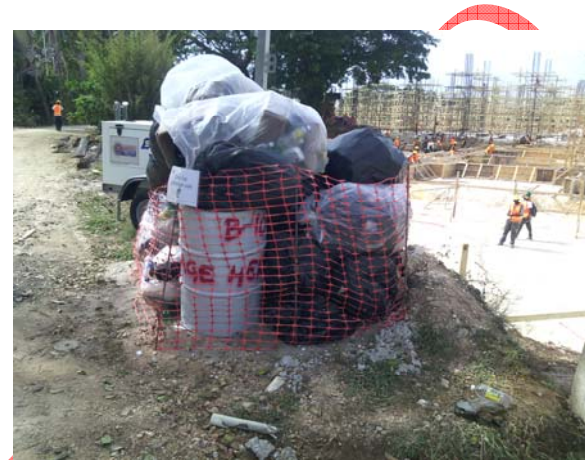
Photo 10: Solid waste stored and bounded off on the site. Several of these were across the property. Photo taken 29 January 2016 by NEPA Officer
