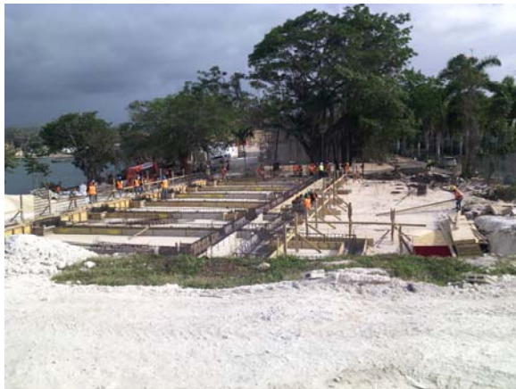
Photo 9: Building 13 at foundation stage. Photo taken 29 January 2016 by NEPA Officer
