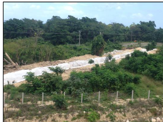
Photo 2: Repaired check dams at K62+400 (Photo taken by NEPA Officer on 10 March, 2016)
