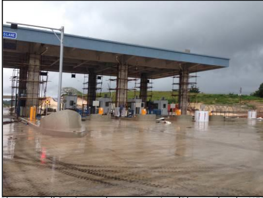
Photo 1: Toll Station under construction (Photo taken by NEPA Officer on 18 February, 2016)
