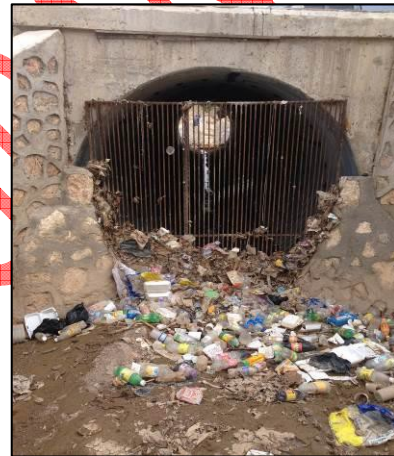
Photo 4: Bar Screen used to cover culvert at the Mammee Bay round about (Photo taken by NEPA Officer on 18 February, 2016)
